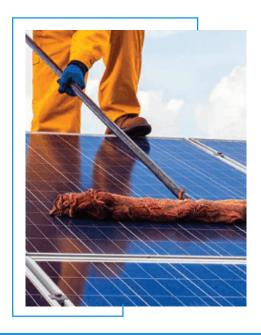
The more light that hits a panel, the more power it will generate. One of main issue with solar panels is the attraction of birds. Bird droppings can also compromise the efficiency of your solar Power system. As Solar Panel is in open areas or rooftop so dust will start to settle on them which block sunlight and start reducing their efficiency. There are different possibilities of efficiency drop when solar panel is not cleaned. Let's have a look on the below table:
